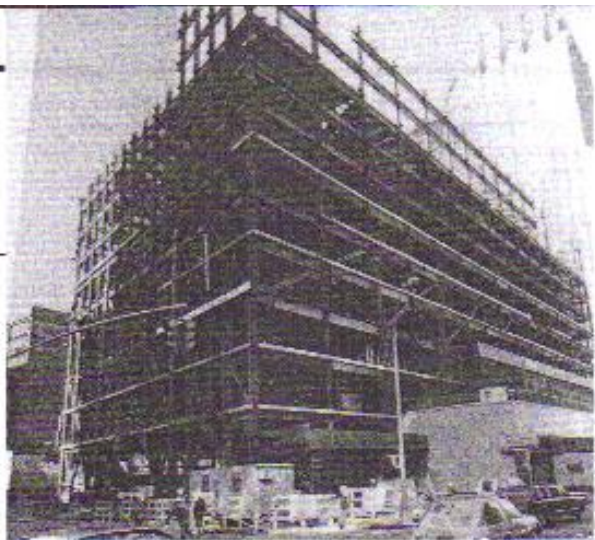
Lower levels with wind truss system tough to build.
